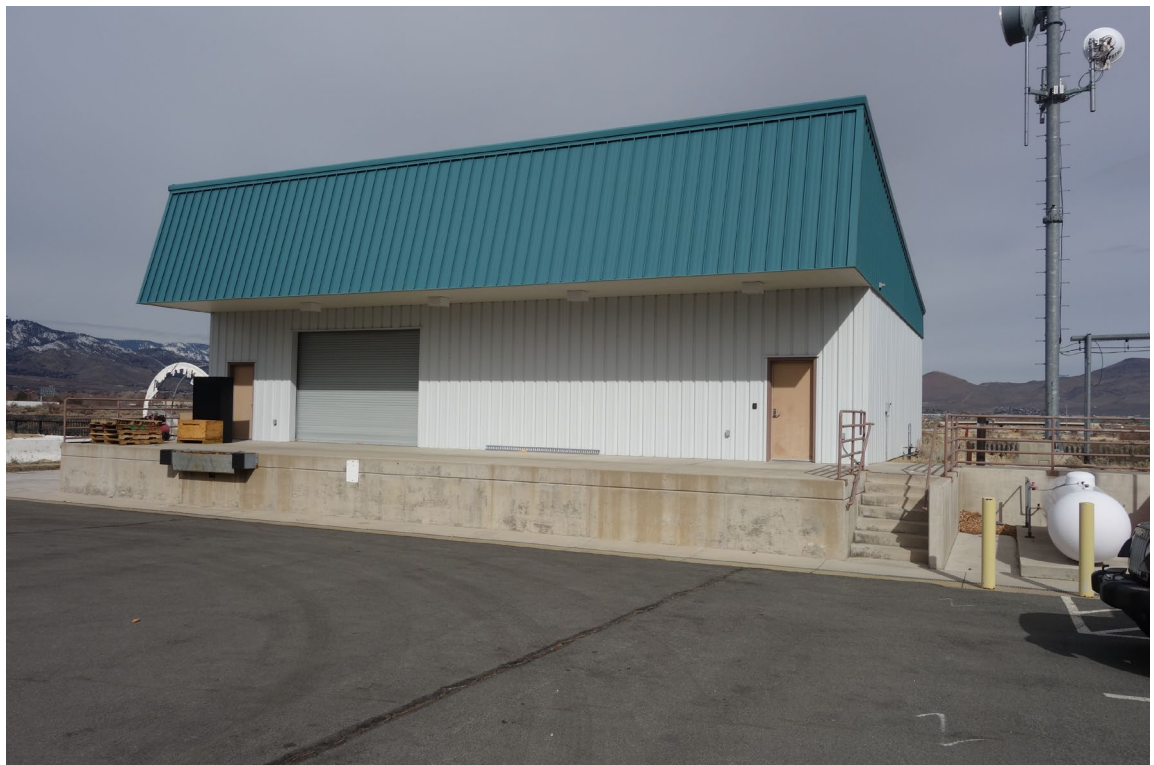
SEOC Warehouse – FCA Building #2914 Description: Exterior View of the Building.
