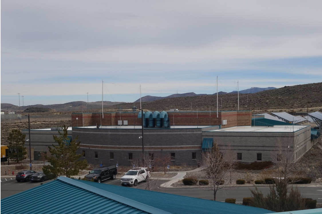
State Emergency Operations Center – FCA Building #2913 Description: Exterior of the Building.
