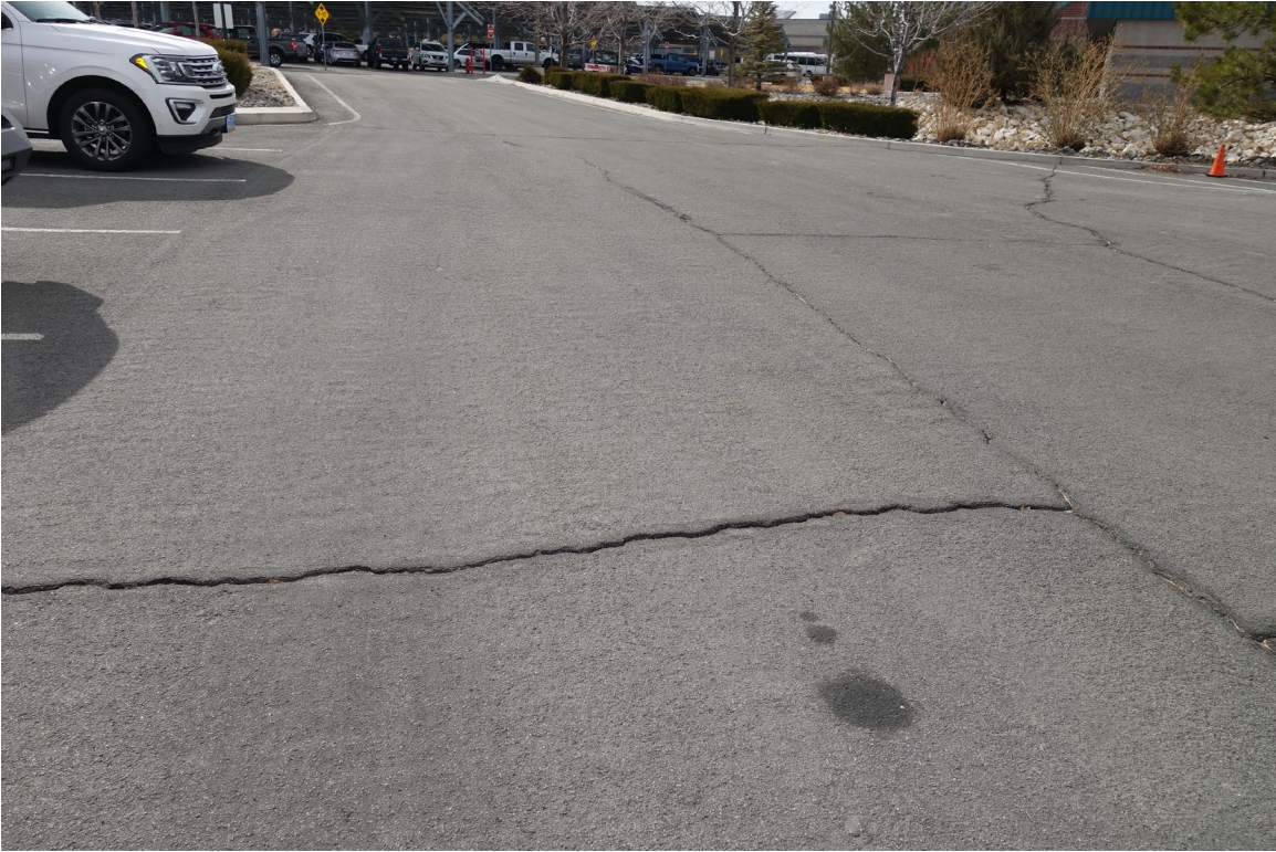
State Emergency Operations Center Site – FCA Site #9816 Description: Crack Fill & Seal Asphalt Paving.
