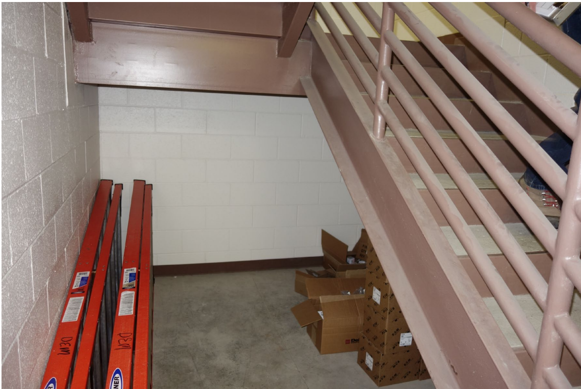
State Emergency Operations Center – FCA Building #2913 Description: ADA Cane Detection Needed.
